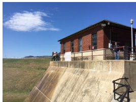
Control House of the Conklingville Dam on the Great Sacandaga Lake
