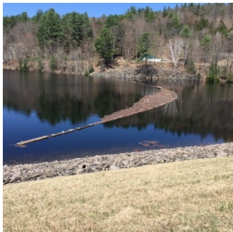
The log boom at the Conklingville Dam prevents debris from going into the spillway and the turbines of the hydroelectric facility
